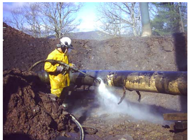
Operator using NLB's NCG8400A-3 Rotating Hand Lance for 100% coating removal.
