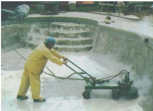
The NLB model 36-1500-20A SPIN JET® is ideal for removing coating on flat surfaces.
