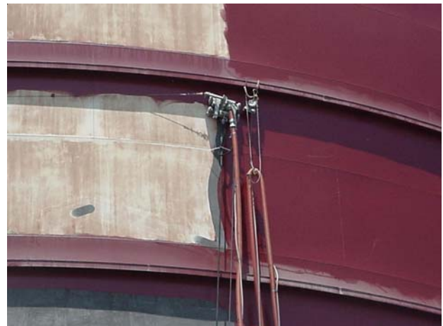
The mobility of NLB's Crawler allows it to get within six inches of an obstruction.
