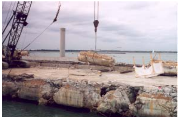
Once the concrete and steel was removed the beams were lifted away with a crane.
